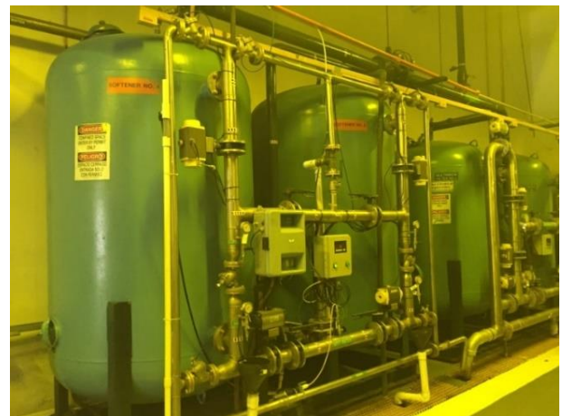
(Fig 3) arrangement of filter tanks and softener
