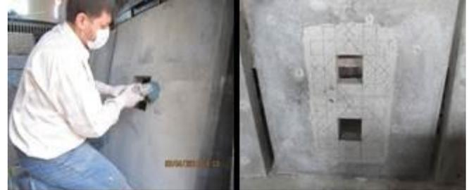
Figure (5) Concrete surface preparation by electrical grinder
