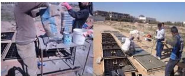
(b) Mixing and casting process
