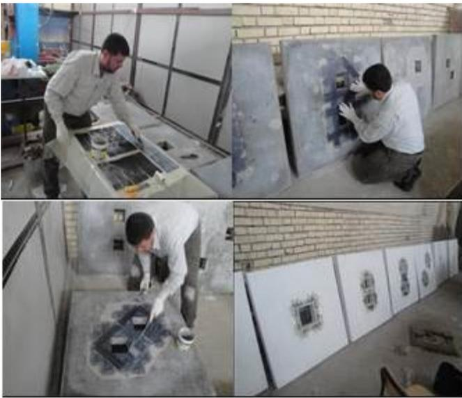
Figure (6) Installation of CFRP sheets
