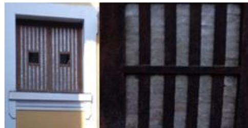
*Fig.6.Oyster shells in window shutters.*
