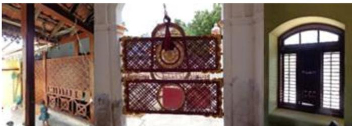
**Fig.8.** Wooden screens in courtyards, balcoes and louvres in the window.
