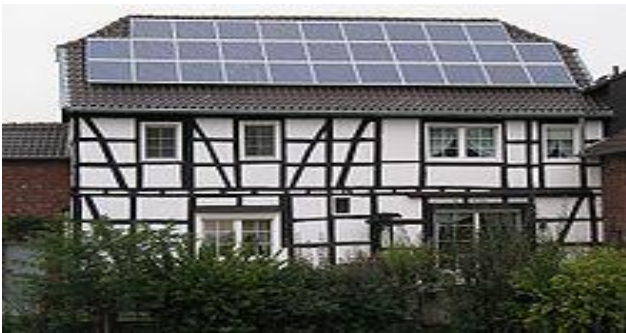
Figure 2.0 Off-Grid Roof Integrated Solar Photovoltaic System
