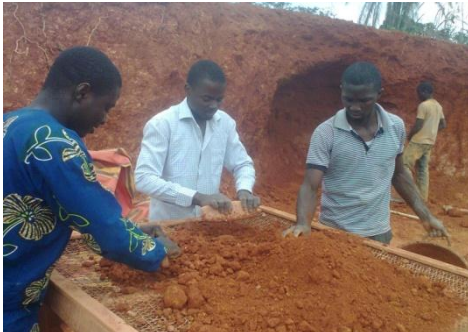
Fig. 1 Screening of Soil through 12mm Wire Mesh
