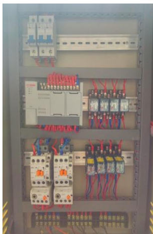
Figure 3.2 Installment of Components on Panel Box
