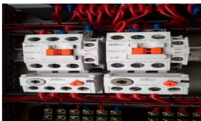
Figure 2.26 TOR connection with MC
