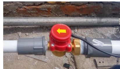
Figure 2.32. Flow Switch
