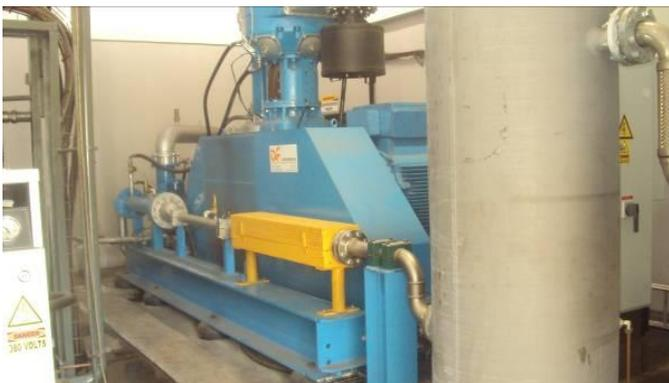
**Figure 13: The 40 bar air compressor in service**
