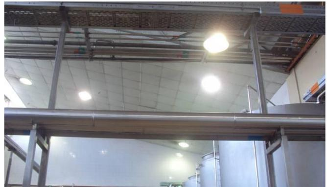
**Figure 10: Unnecessary lighting during the day**
