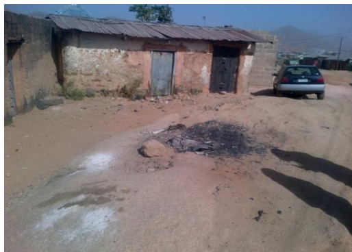
Plate 2: A dilapidated building in one of the selected slums
