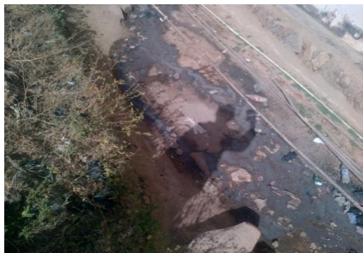
Plate 3: Water pipe going through contaminated water in one of the slums
