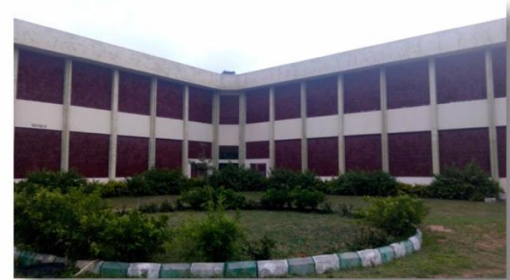
Figure 1.9 showing integrated shading at the south elevation Source: Physical Survey
