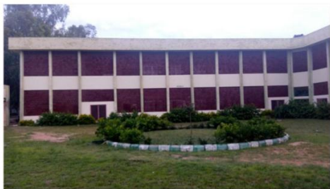
Figure 1.8 showing integrated shading at the south elevation Source: Physical Survey
