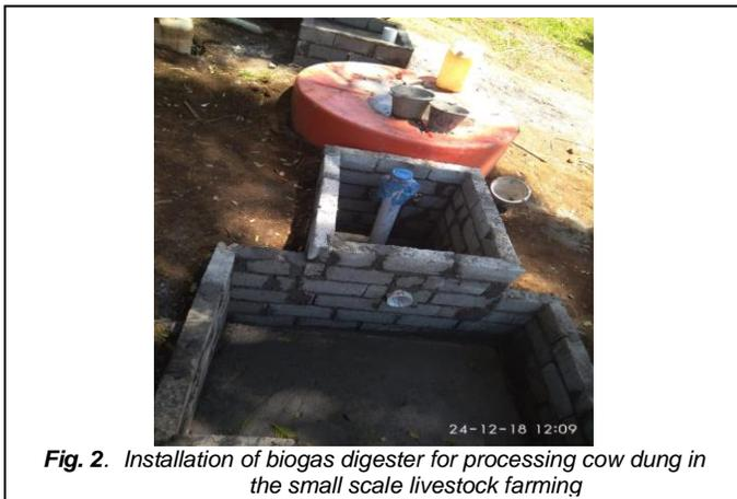
**Fig. 2.** Installation of biogas digester for processing cow dung in the small scale livestock farming
