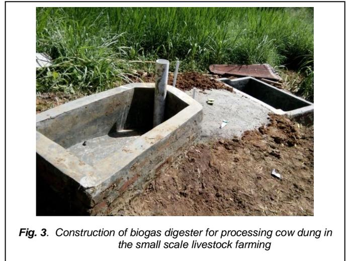
**Fig. 3.** Construction of biogas digester for processing cow dung in the small scale livestock farming
