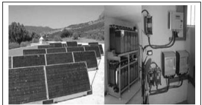
Fig. 2. A dc PV-diesel hybrid system with 8kwp PV, 20kVA-diesel, 48 @1500Ah battery and 16kw inverter power for home users in Spain [10]
