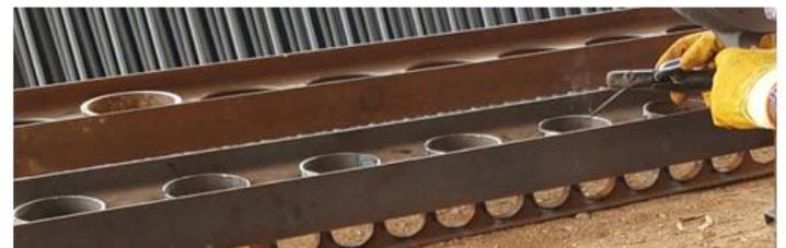
*Fig.(4). Installation Of Ring Stiffeners*
