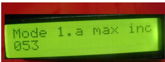
Fig 20: Display of Maximum temperature of the room set by the user at the Transmitter Section
