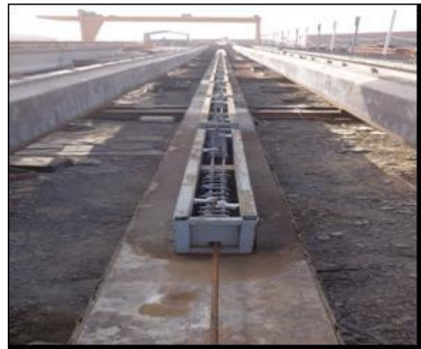
Figure(8) Pulling of Steel Strand Before Casting
