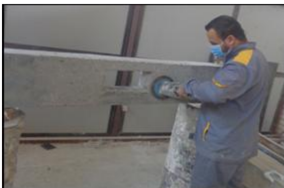
Figure (10) Concrete Surface Preparation by Electrical Grinder.
