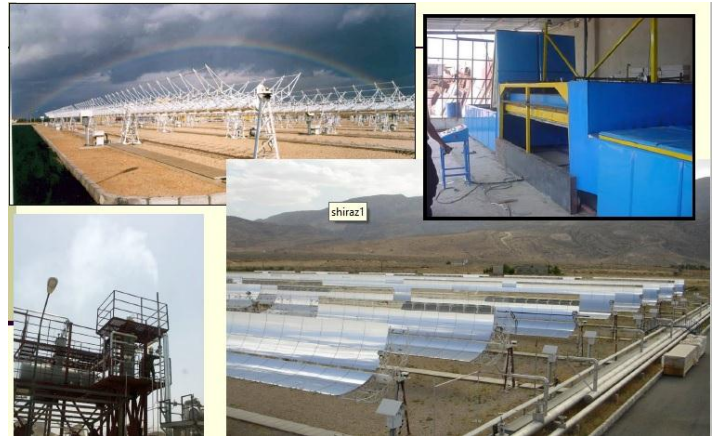
Fig. 11. Shiraz 250 KV Parabolic Trough solar thermal power plant
