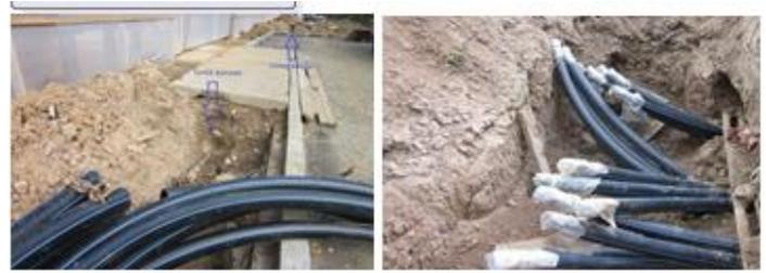
**Fig 4.** Route and methods of laying heating networks.
