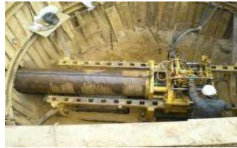
*Fig 1. Pipe laying by manual punching.*
