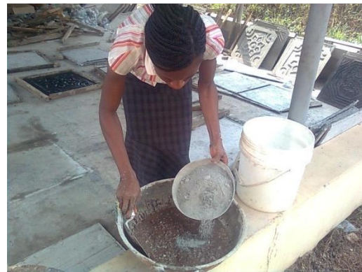
Mixing of sharpsand, with cement
