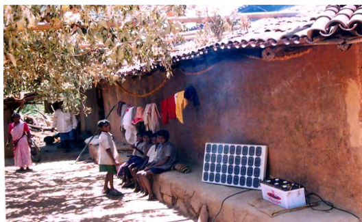
Fig 9 : Solar Home Lighting system in a village house
