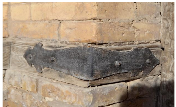
Fig. 4. a) The General view of wooden bars with metal elements. Islam Khoja madrasah (Khiva)
