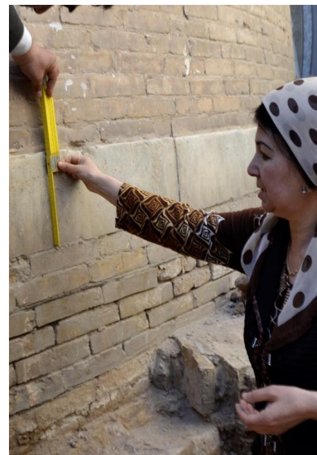
b) seismic isolation from marble block
