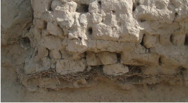
Fig. 4. b) The General view of wooden bars with metal elements. Nazlumkhan suluw mausoleum (Khojeyli city)
