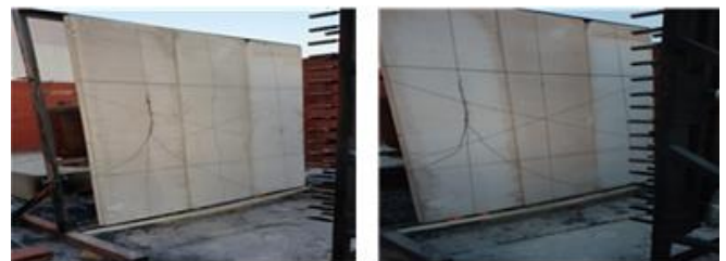
Fig. 11. Photographs of a firewall(ALC) before and after experiments.
