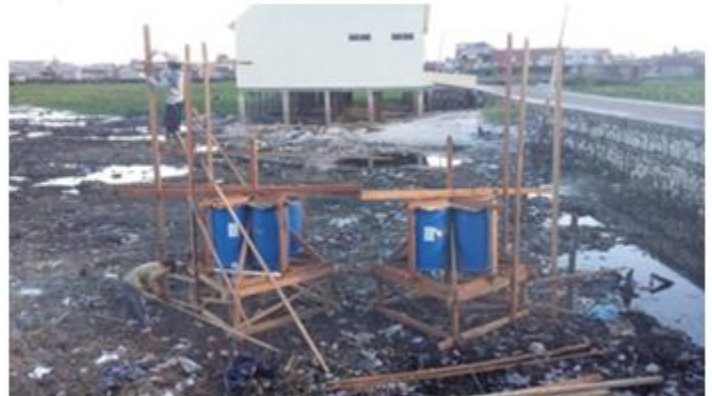
Fig 2. The Trial Construction and the Assembling Process
