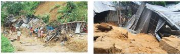
Figure 1 View of Landslide in Chittagong
