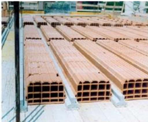
Fig.1.2 Inverted T-beam
