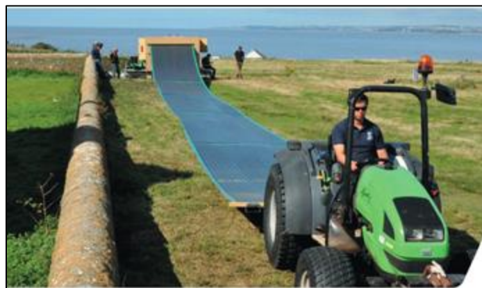
Figure 2: Rapid Roll unfurling solar arrays like a carpet from behind a truck [2]
