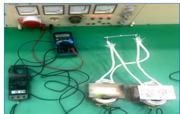
Figure (8): Two transformers connected to the power supply with parallel and short circuit
