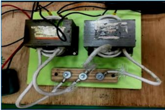
Figure (9): Two transformers connected to the power supply with series and short circuit
