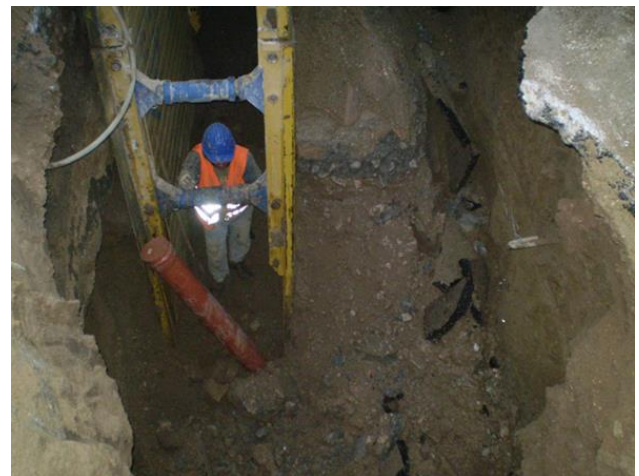
Fig. 5. Worker protection within support, Larissa, Greece, 2012 [15].
