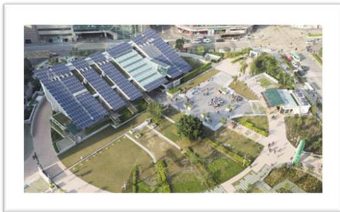
Fig. 4: Onsite installed Solar PV Panels
