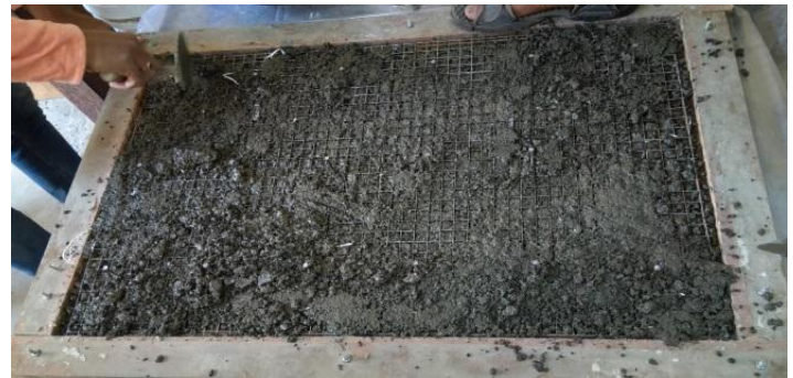
Figure 4.1 Casting of Ferrocement Panel
