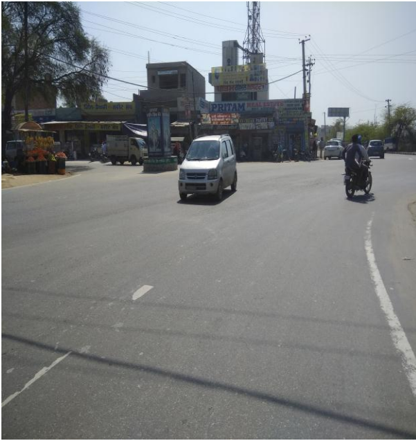
Fig 5: Improper Junction Design
