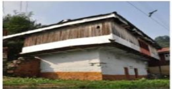
Figure .1 Kath-Kunni Construction view
